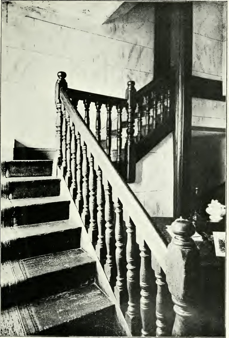
STAIRCASE AT GARSDON MANOR HOUSE. (Lower Portion.)
